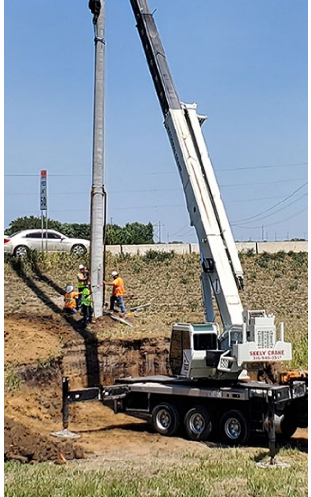
A pole for a new camera is installed along I-235 in Wichita as part of providing traffic information for WICHWay. Photo by Tracy Crockett, District Five
